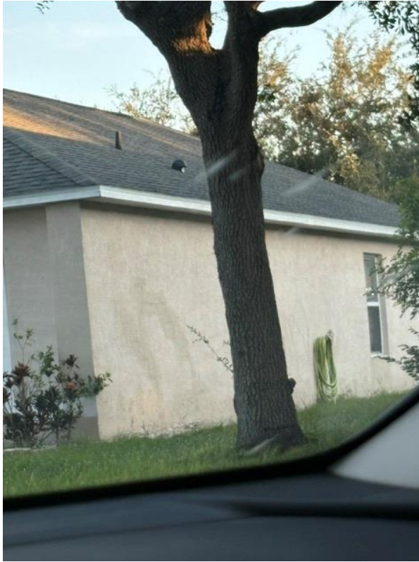
Exterior paint conditions
