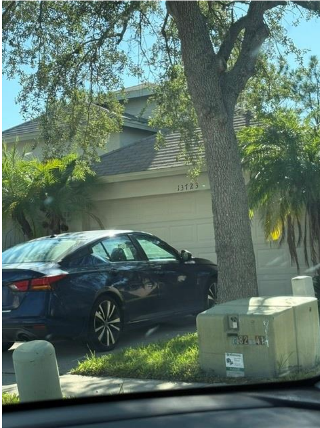
13723 Ogakor lack of tree maintenance (palms & oaks)
